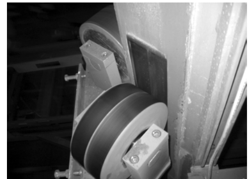
Floor-to-floor elevator guide wheel of NYTEC-HS
